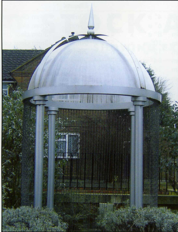
WATER FEATURE - ALL SAINTS CHURCH, WATFORD The water rises up the pillars & runs out over the DOME into the reservoir below.
